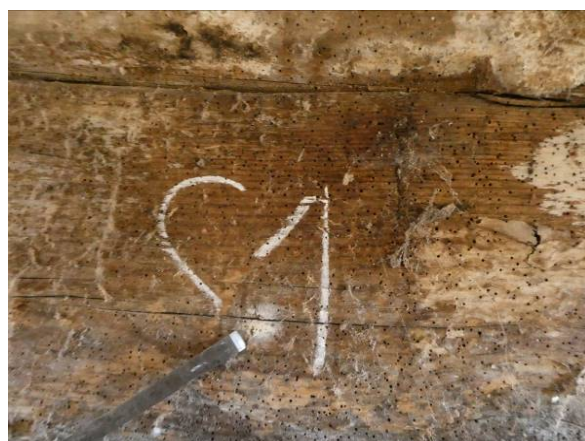
Obr. 11 – Črvotoč v prievlaku C1, +2,800m - detail
